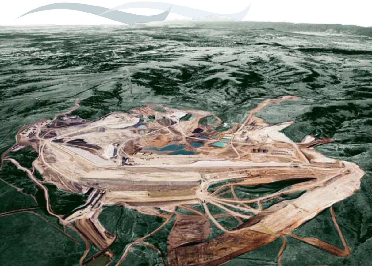
[ Rueter-Hess Reservoir under construction ] Photo: Jackie Schumaker Photography
